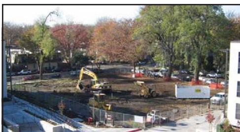
Construction underway at Fremont Community Garden.
